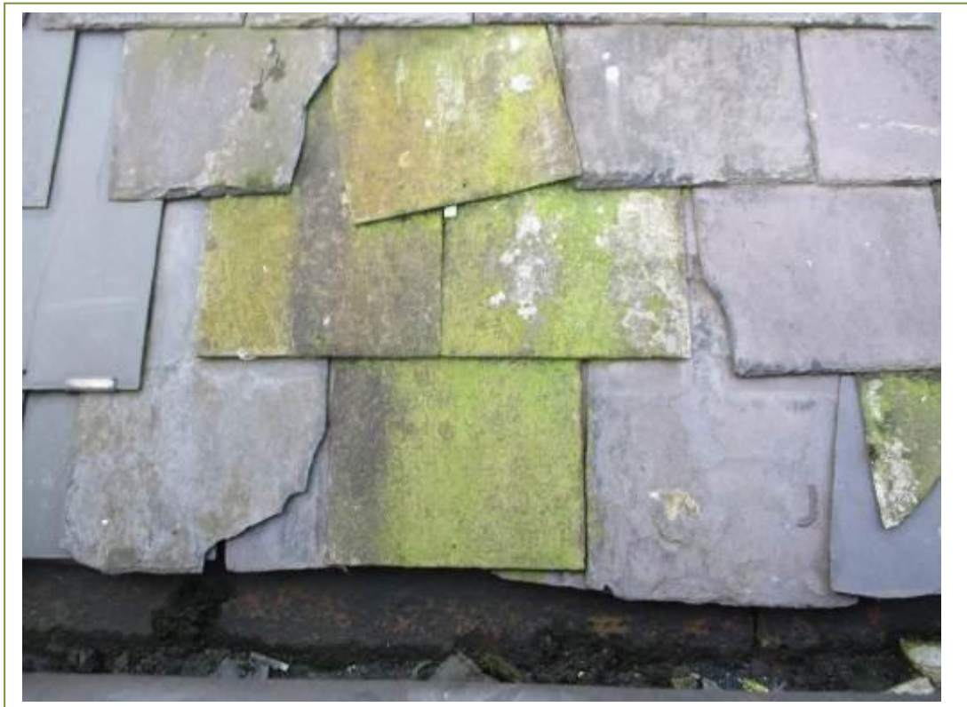
Cement replacement slates identified on the rear roof beside the main pitched roof
