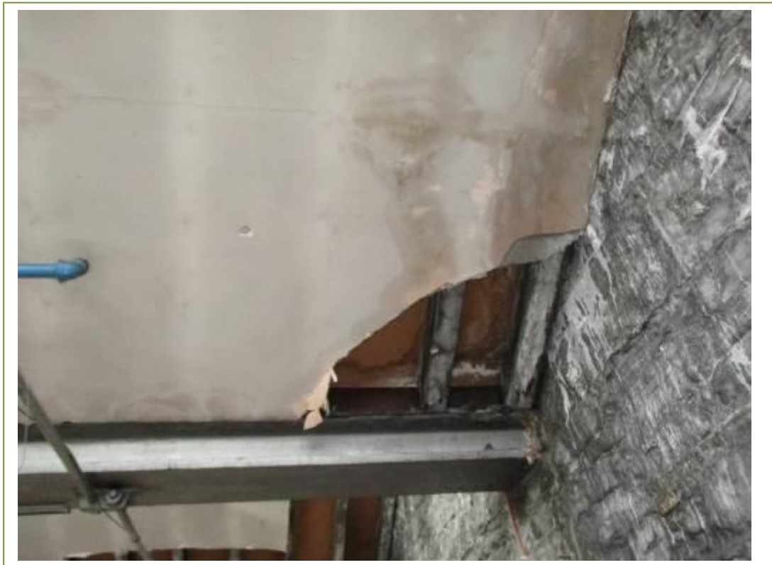
Plasterboard ceiling boards under main pitched roof. No ACM's detected
