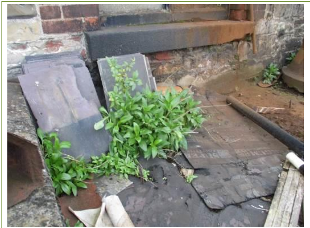
Cement slates identified on the flat roof area
