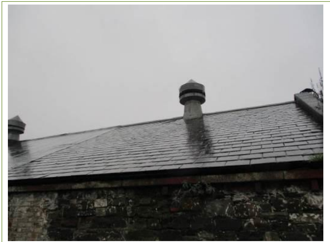
Natural slates on some rear roofs. No ACM's detected
