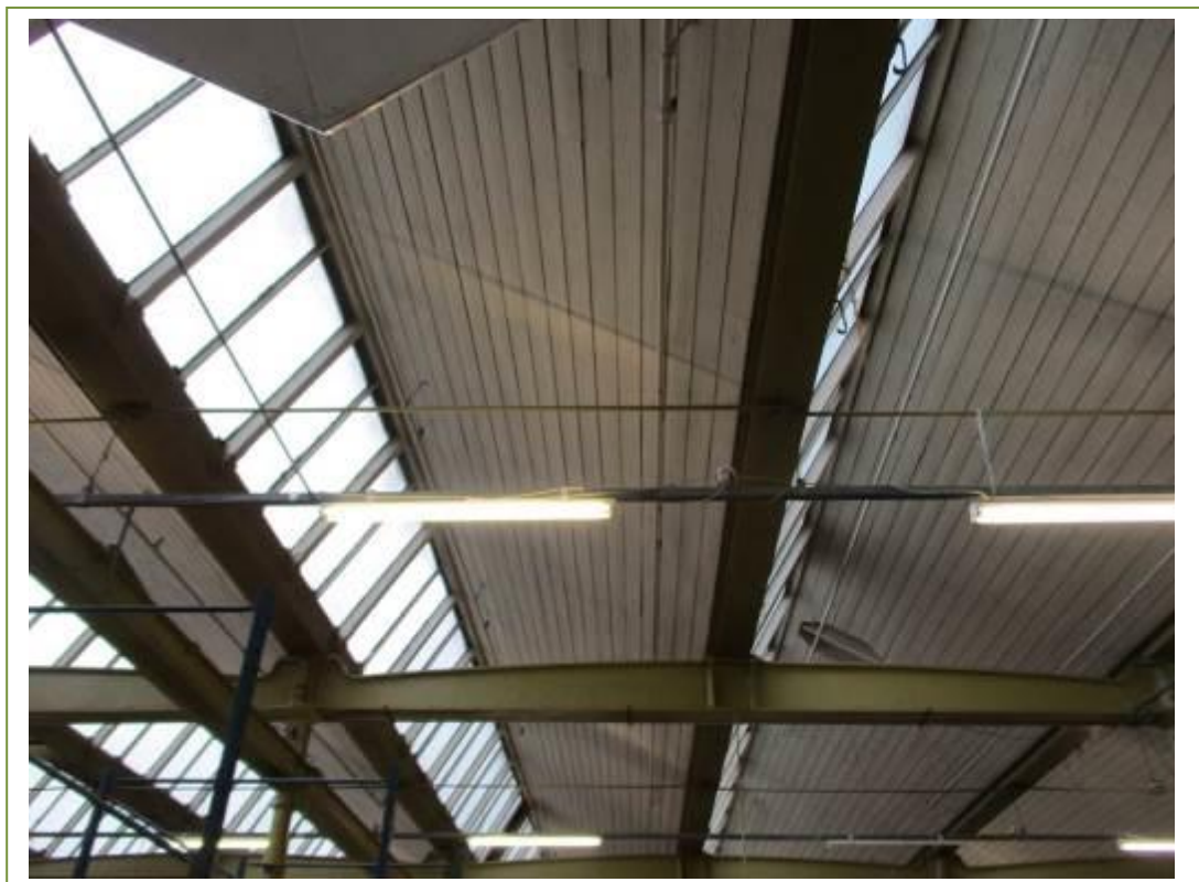
View of the lining boards under the felted pitched roof
