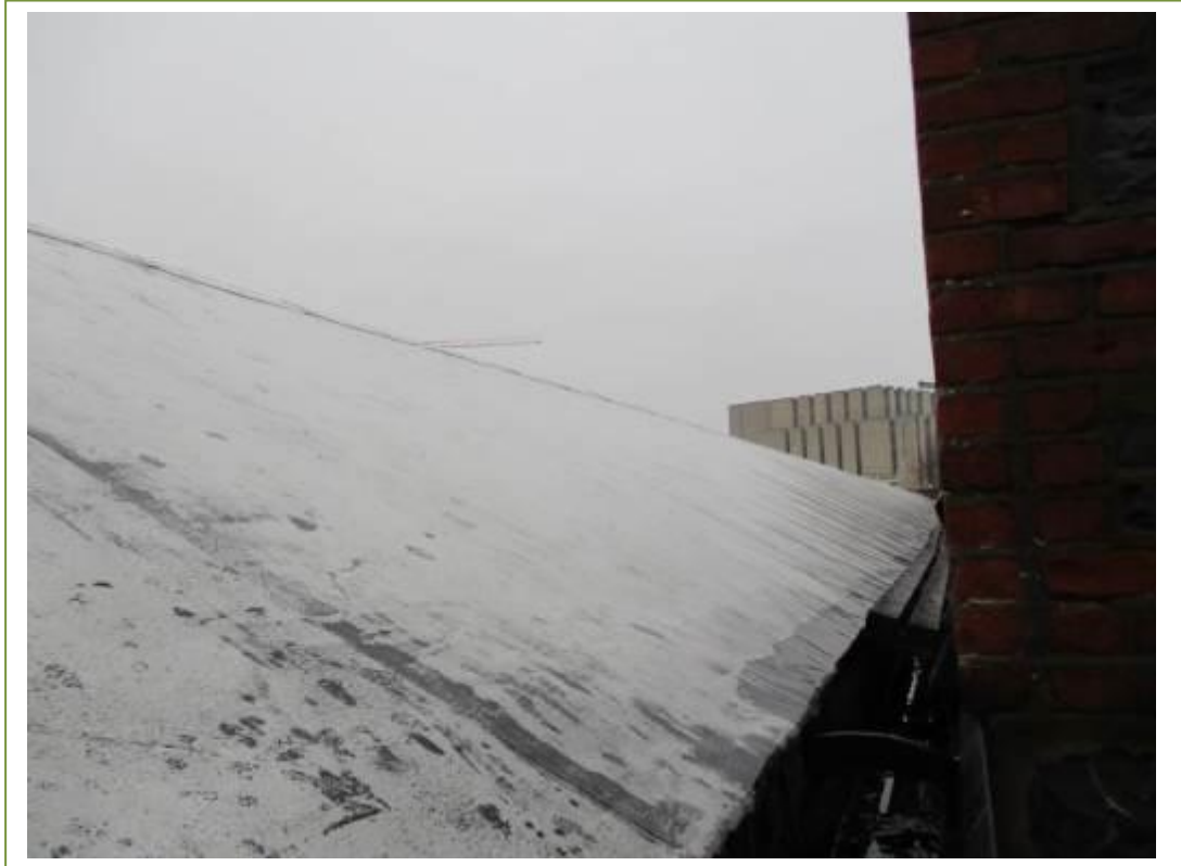
Felt on main pitched roof. No Asbestos Containing Materials (ACM's) detected
