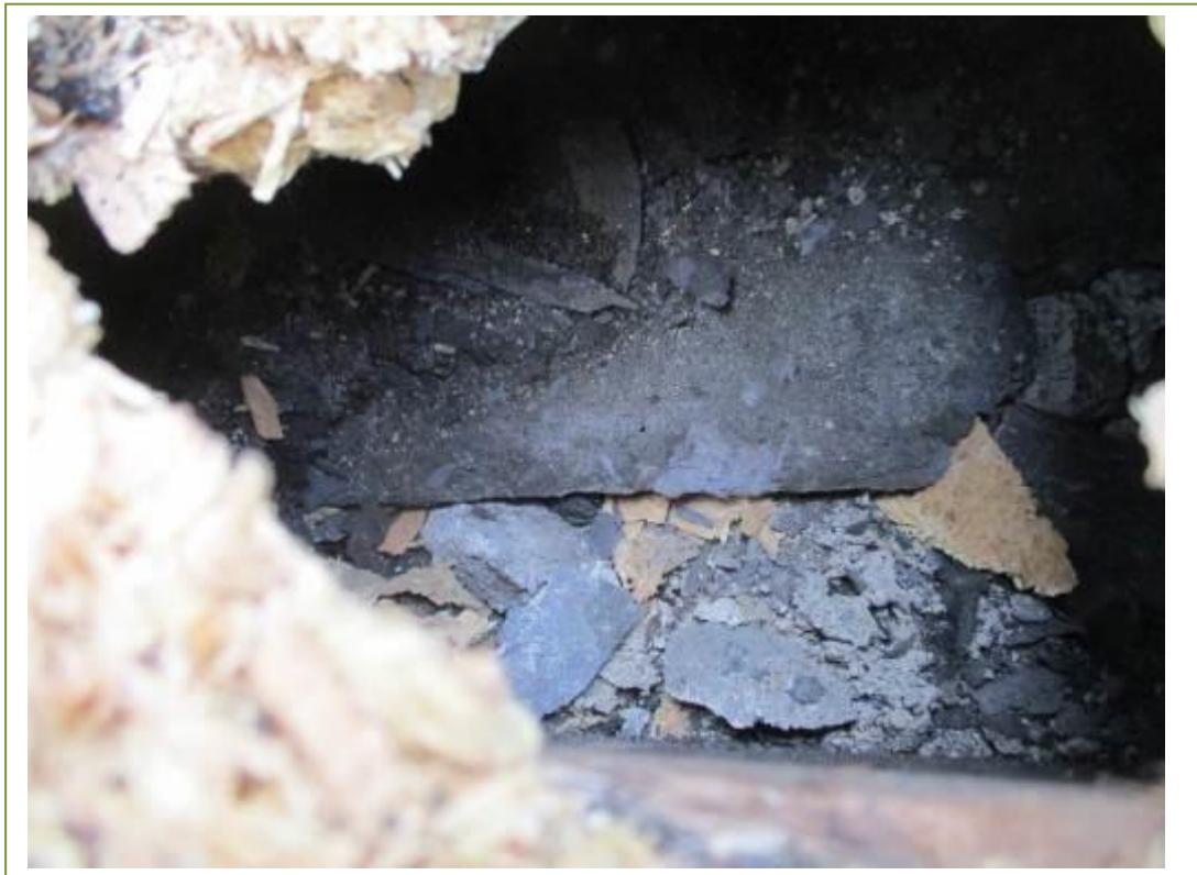
Natural slates present in the void between the felted roof and the lining boards beneath
