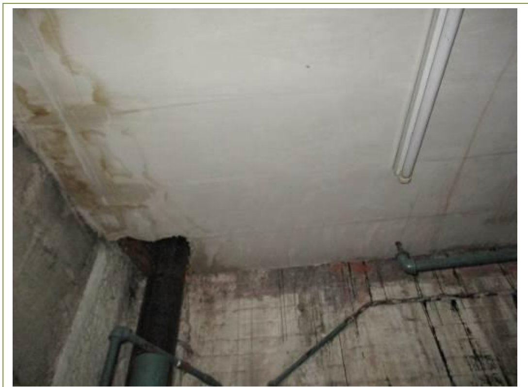
Plasterboard ceilings in sprinkler room. No ACM's detected
